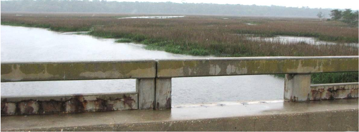
Figure A.3: Corrosion Damage in Cast-in-Place Barrier of Harriett's Bluff Road at Deep Creek Bridge (Bridge No. 039-0049)
