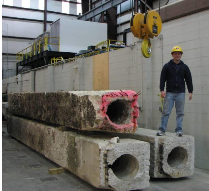
Figure 3.5: Piles from Turtle River Bridge
