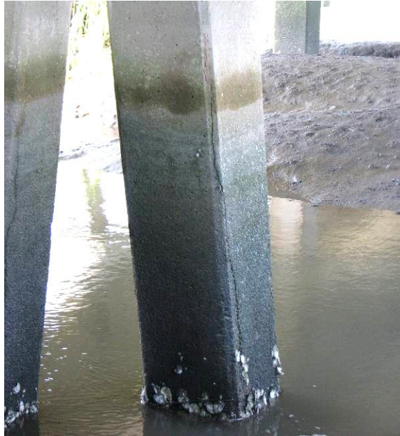
Figure A.8: Vertical Cracking at Corner of Concrete Pile on US 17 at Back River Bridge (Bridge No. 051-0059)
