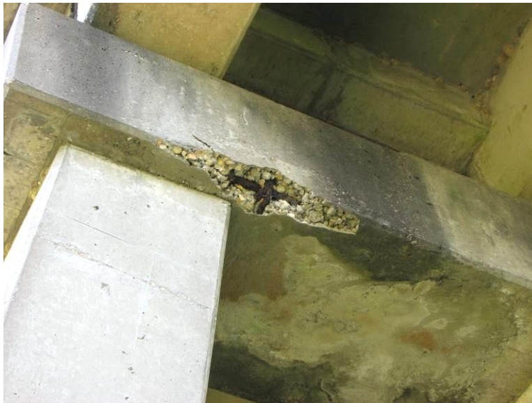
Figure A.12: Honeycombing and Exposed Corroding Reinforcement in Pile Cap on US 80 at Lazeratto Creek Bridge (Bridge No. 051-0066)
