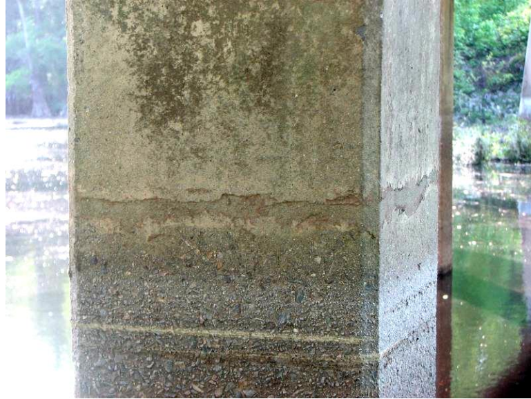
Figure A.19: Grout Repair of Transverse Cracking Likely Caused by Overdriving on Long Bridge Road at Ebenezer Creek Bridge (Bridge No. 103-0030)
