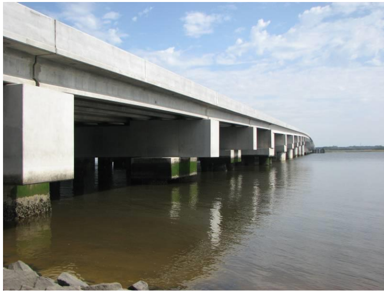
Figure A.21: Updated I-95 at Turtle River Bridge (Bridge No. 127-0052)
