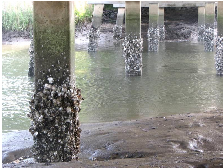
Figure A.17: Pile-Bent Substructure of Oatland Island Research Bridge (Bridge No. 051-5013)
