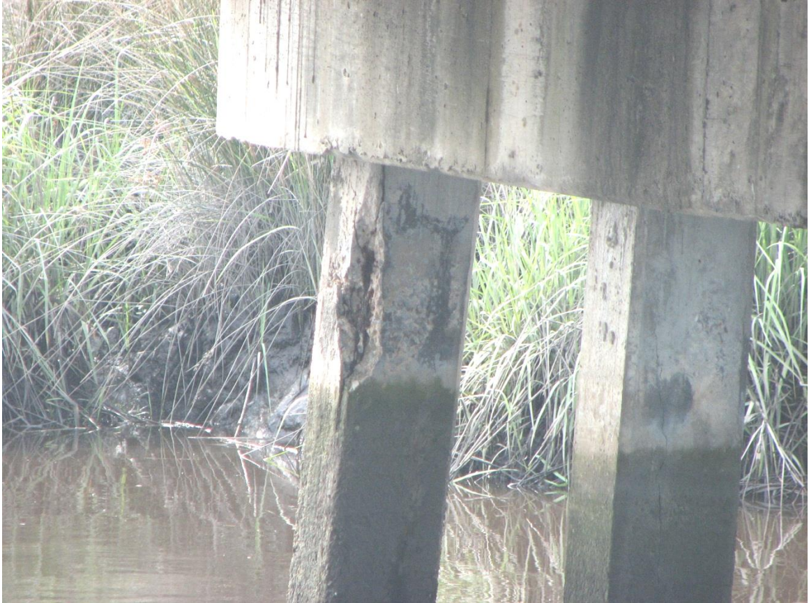
Figure A.27: Deterioration of Precast Concrete Piles in Substructure of Ocean Highway at Riceboro Creek Bridge (Bridge No. 179-0005)
