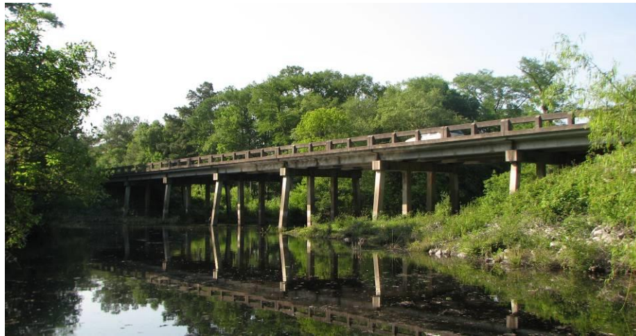
Figure A.18: Long Bridge Road at Ebenezer Creek Bridge (Bridge No. 103-0030)
