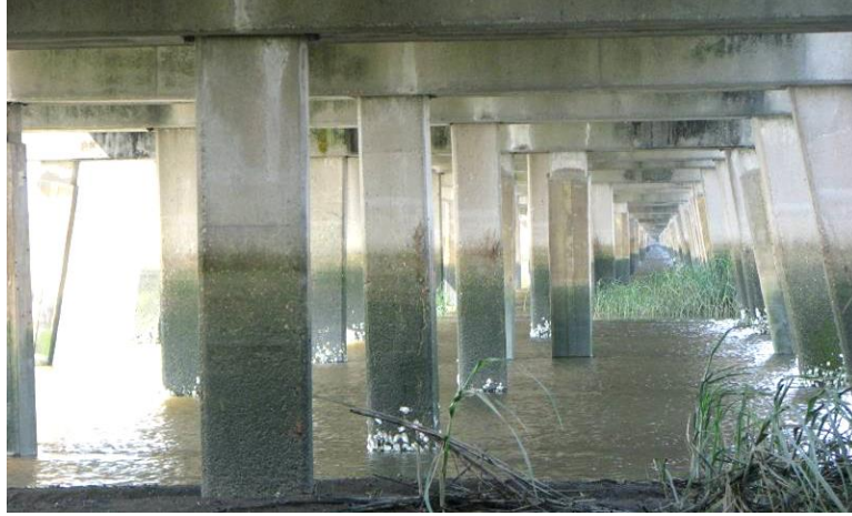
Figure A.7: Pile-Bent Substructure of US 17 at Back River Bridge (Bridge No. 051-0059)
