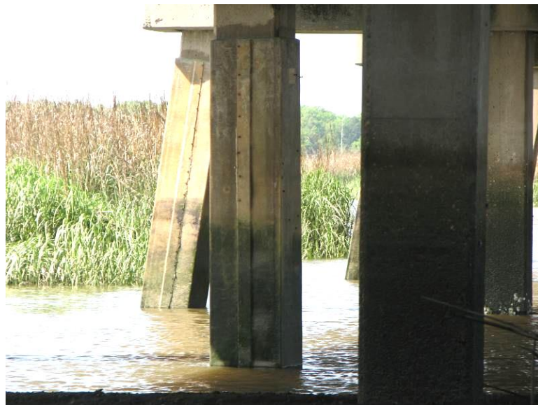
Figure A.9: Corrosion Damaged Piling with FRP Jacket Retrofit on US 17 at Back River Bridge (Bridge No. 051-0059)
