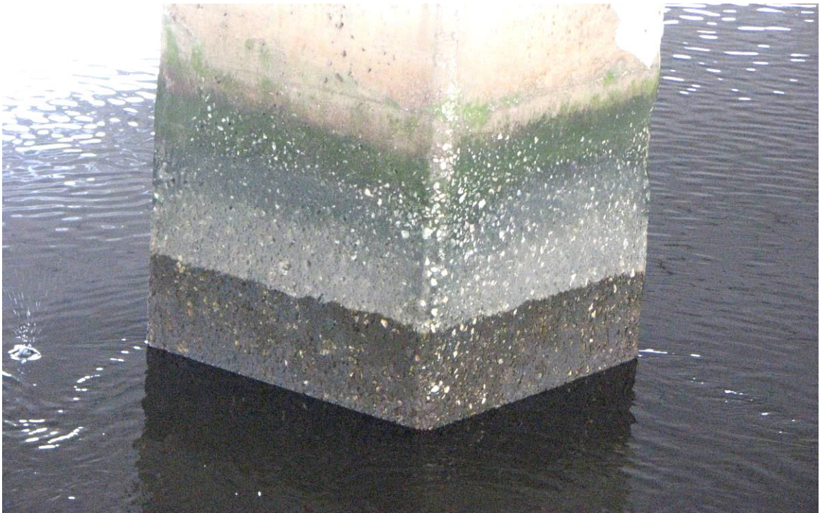
Figure A.30: Typical Surface Abrasion of Concrete on Ocean Highway at Champney's River Bridge (Bridge No. 191-0005)
