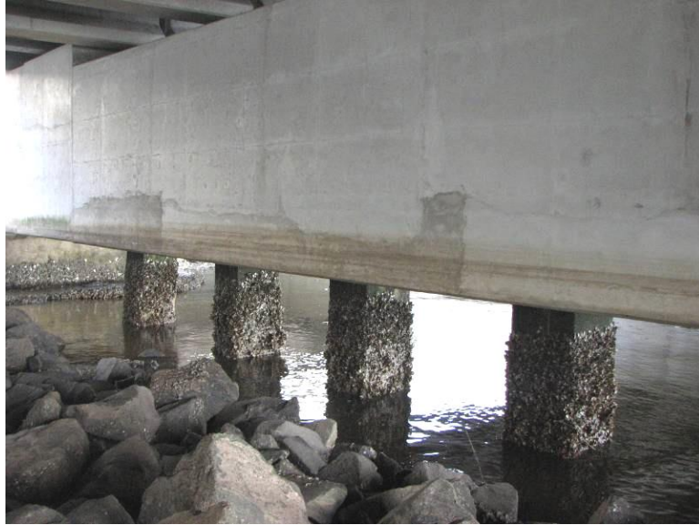
Figure A.22: Transfer Beam with Original Piles Left In-Place on I-95 at Turtle River Bridge (Bridge No. 127-0052)
