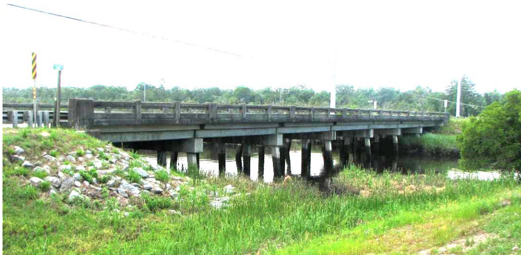
Figure A.26: Ocean Highway at Riceboro Creek Bridge (Bridge No. 179-0005)
