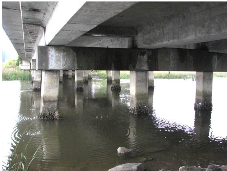
Figure A.2: Substructure of Harriett's Bluff Road at Deep Creek Bridge (Bridge No. 039-0049)
