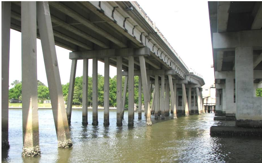
Figure A.13: Underside of Island Expressway at Wilmington River Bridge (Bridge No. 051-0132)
