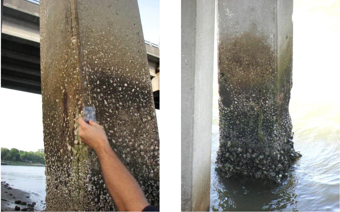
Figure A.15: Severe Damage to Concrete Piling on Island Expressway at Wilmington River Bridge (Bridge No. 051-0132)
