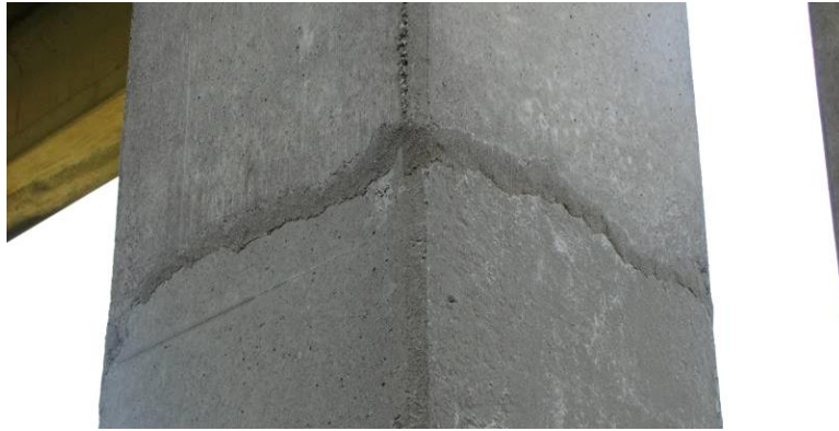
Figure A.11: Grout Repair of Traversve Crack in Precast Concrete Pile on US 80 at Lazeratto Creek Bridge (Bridge No. 051-0066)
