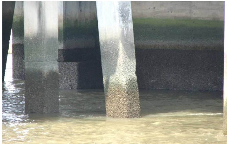
Figure A.5: Surface Abrasion of Concrete Substructure on Houlihan Bridge (Bridge No. 051-0054)
