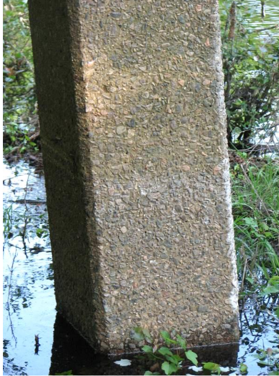
Figure A.20: Surface Abrasion of Concrete Below High-Water Mark on Long Bridge Road at Ebenezer Creek Bridge (Bridge No. 103-0030)
