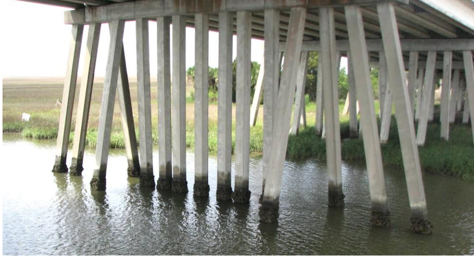
Figure A.24: Pile-Bent on Torras Causeway at Little River Bridge (Bridge No. 127-0063)
