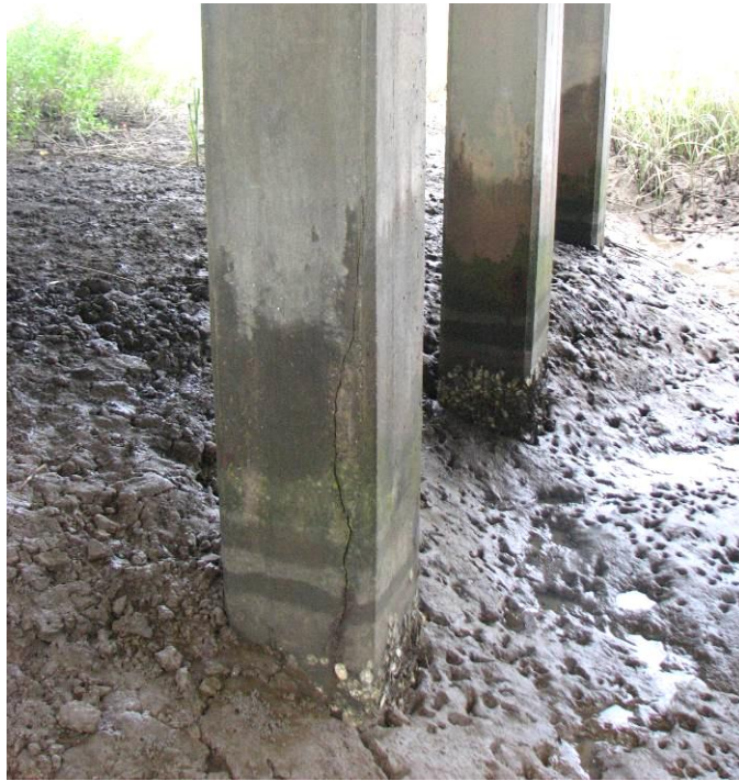
Figure A.25: Corrosion Damage in Original Torras Causeway at Little River Bridge
