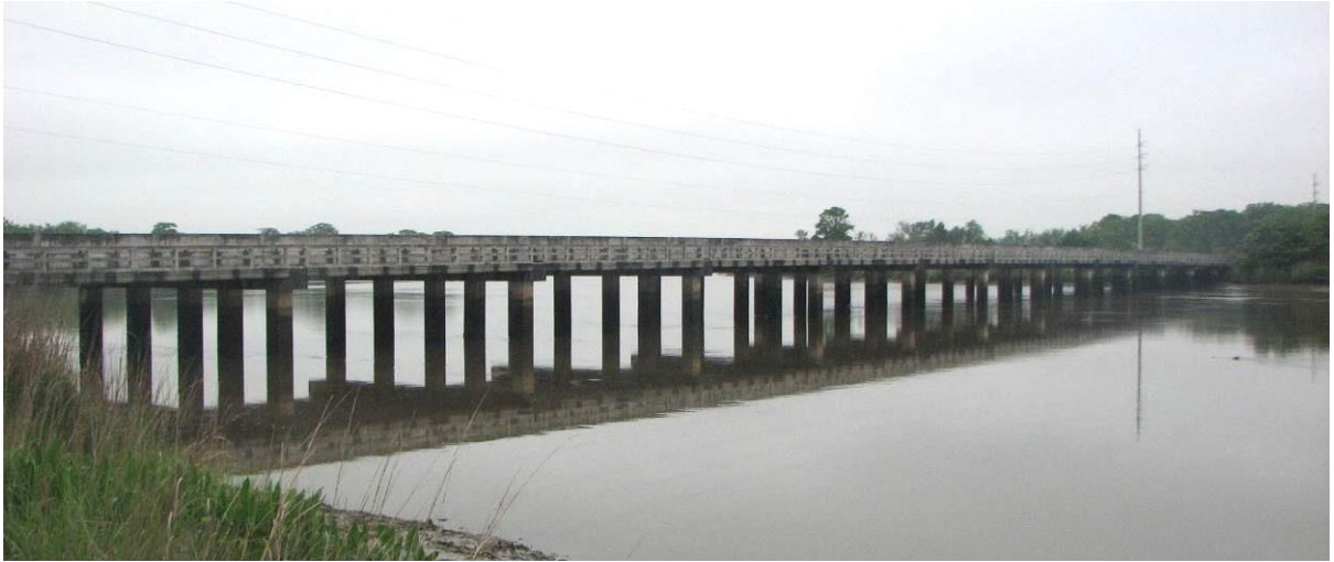
Figure A.28: Overall View of Ocean Highway at Champney's River Bridge (Bridge No. 191-0005)
