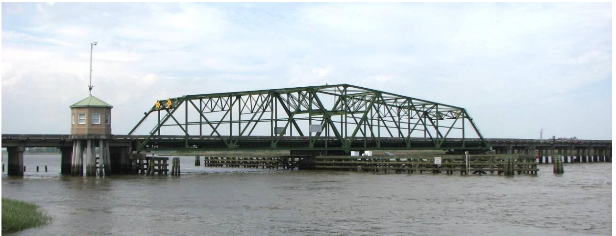
Figure A.4: Overall View of Houlihan Bridge (Bridge No. 051-0054)
