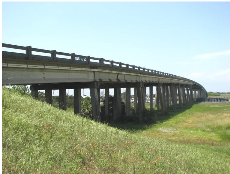
Figure A.10: Overall View of US 80 at Lazeratto Creek Bridge (Bridge No. 051-0066)
