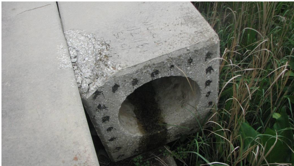
Figure A.29: Remaining Piles on Bank Adjacent to Ocean Highway at Champney's River Bridge (Bridge No. 191-0005)
