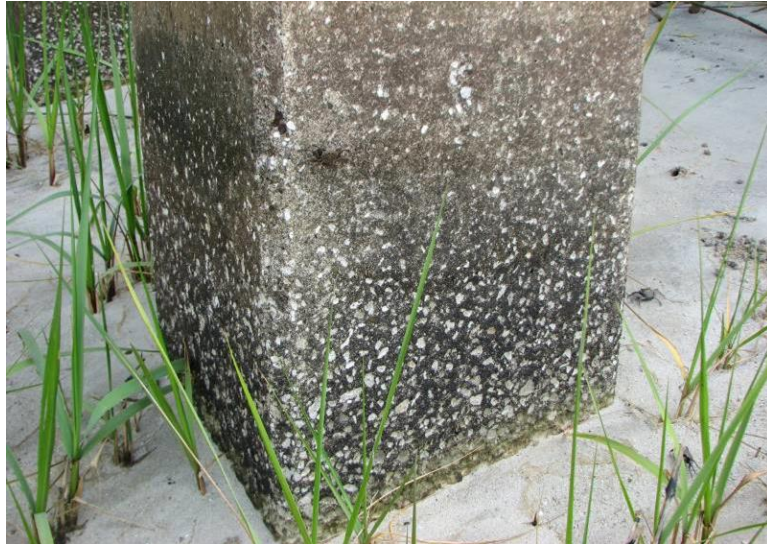
Figure A.14: Deterioration of Limestone Aggregates Present at Concrete Surface on Island Expressway at Wilmington River Bridge (Bridge No. 051-0132)
